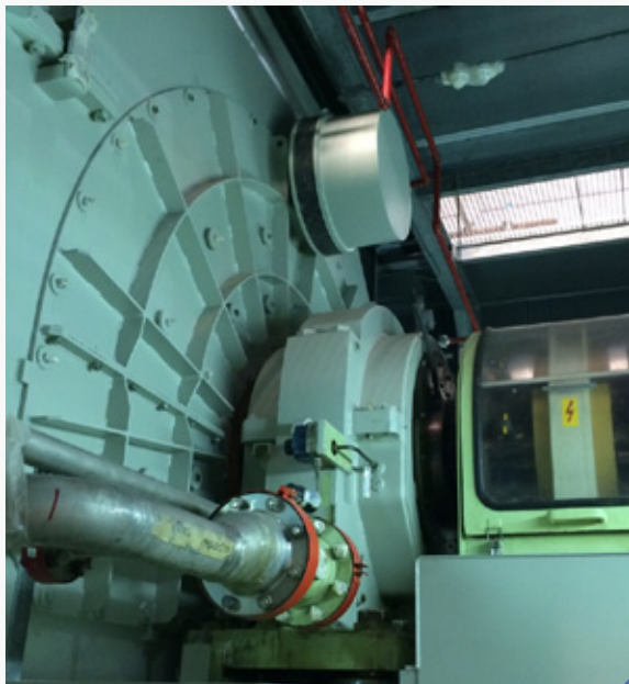
STEAM TURBINE GENERATOR (STG-1) PAINTING AT SOHAR POWER & DESALINATION PLANT
