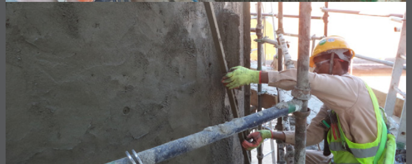
FIREPROOFING WORK AT SOHAR REFINERY INDUSTRIAL PLANT
