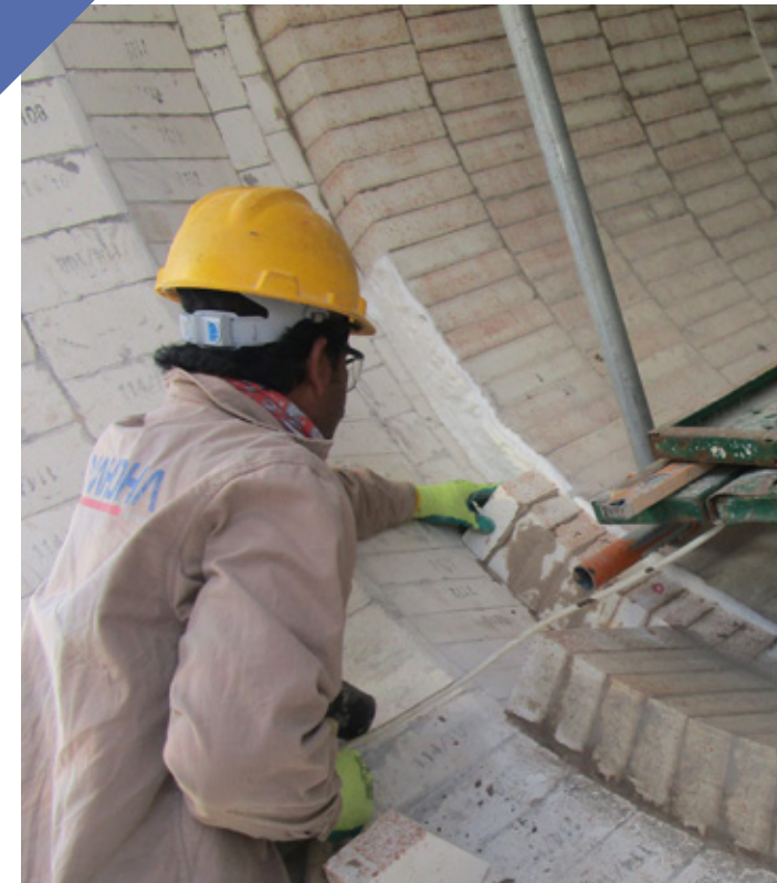
DENSE BRICK LINING IN INCINERATOR AT YIBAL KHUFF
